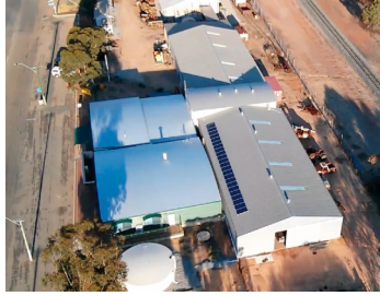
Above - New Solar Panels
